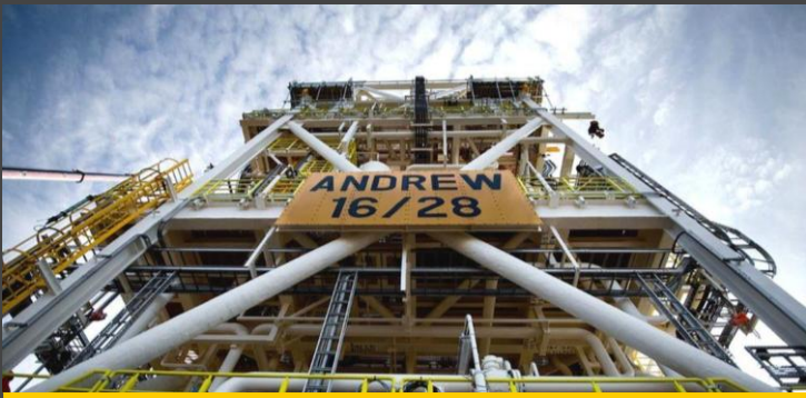
Andrew platform End-to-End Decommissioning
